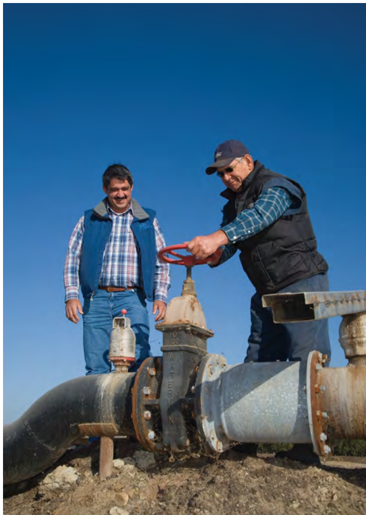
NRCS conservationists monitor a flow meter and gate valve at a dairy in California. The flow meter helps manage nutrients on the dairy.
